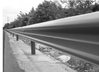
图1 透气型粉末涂料应用于高速公路热浸镀锌喷塑护栏照片 Figure 1 Photo of gas-permeable powder coating applied to freeway's hot-dip galvanized plastic sprayed guardrail
